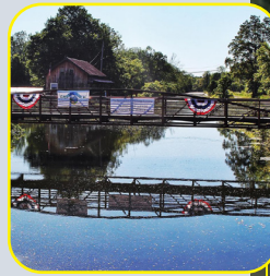
Pedestrian Bridge at Chittenango Landing Museum
