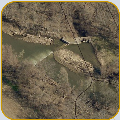
Chittenango Feeder weir and sluice gate
