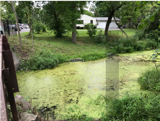
The Chittenango Creek Canal Feeder has diminished flow and becomes stagnant
