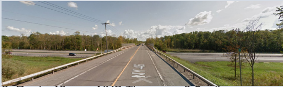
2- Route 46 over NYS Thruway - 0.5 miles
