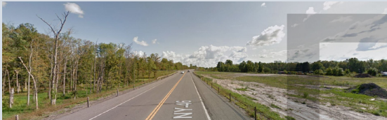
3- Route 46 at Cobb Street - 0.7 miles
