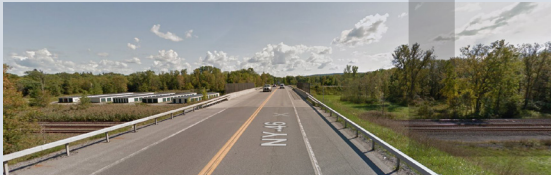
4- Route 46 over CSX Railroad - 0.9 miles
