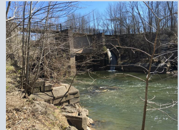
Oneida Creek Aqueduct from Oneida Creek
